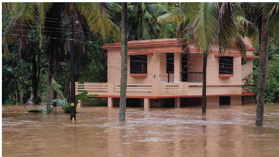
A home at Companypady flooded during 2018 Kerala floods
