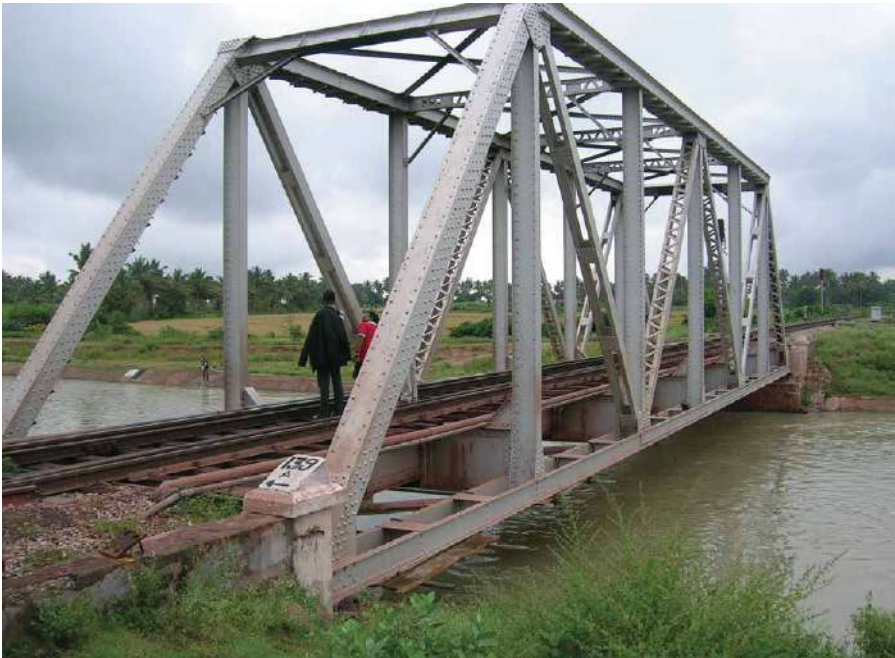
Truss bridge outside Hospet station with a displacement gauge mounted to measure the deflection as the train passes
