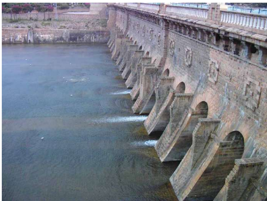
The Krishna Raja Sagara dam beside the Brindavan gardens in Karnataka, India
