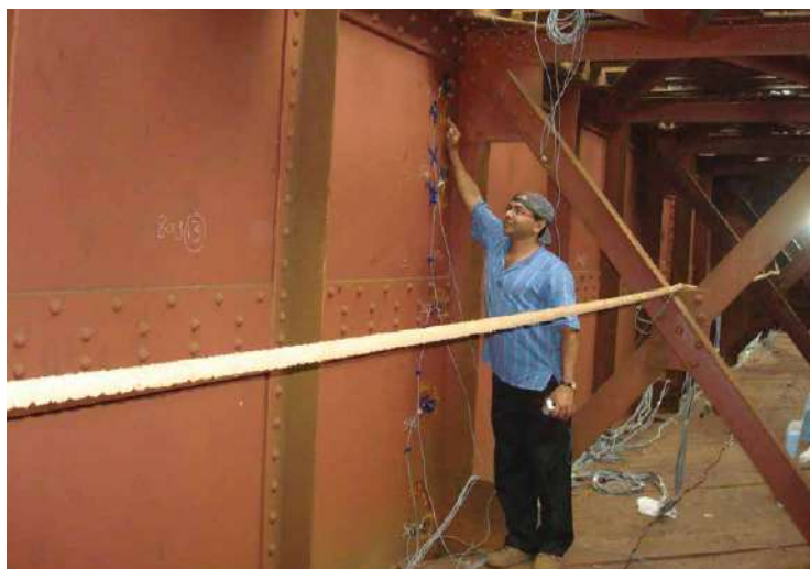
Chandra Kishen at the site of the Escarpment Viaduct Bridge 102 in Braganza Ghats, a plate girder bridge with sensors mounted inside
