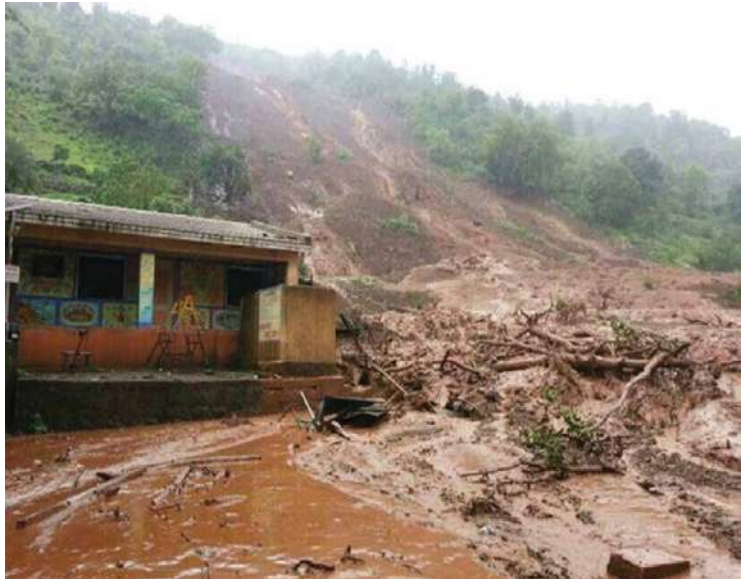
Landslide in Malin village in Pune district, Maharashtra in 2014, resulting in the washout of the village and death of about 150 persons
