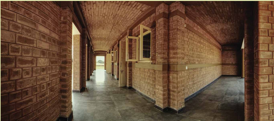
Classroom walls built with stabilised Compressed Earth Blocks (CEB)
