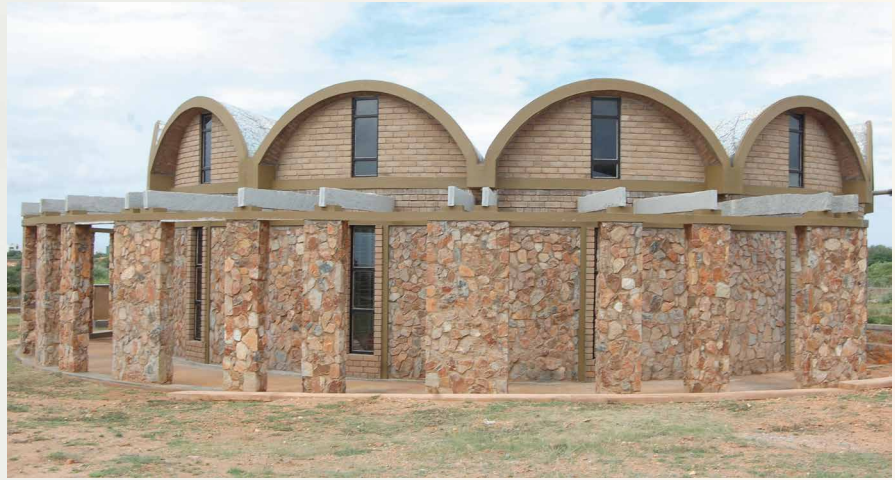
The exhibition centre built with Rubble Rock Masonry (RRM) technique
