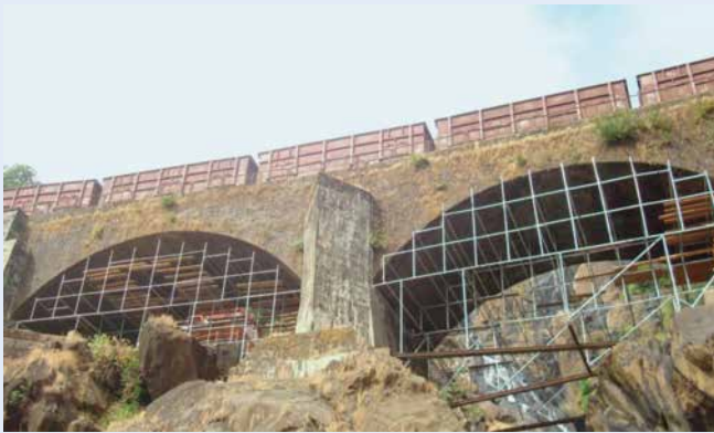
Testing of the Dudhsagar bridge near Goa with loaded railway wagons
