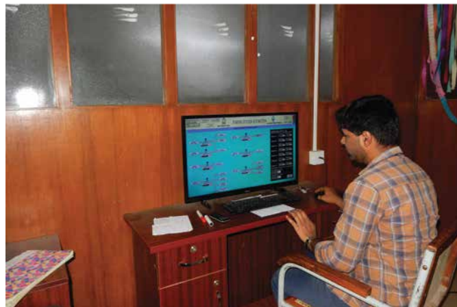
The centralised control room where water levels at various pump houses are monitored
