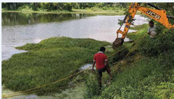
Weed being lifted using JCB, leaving behind clean water
