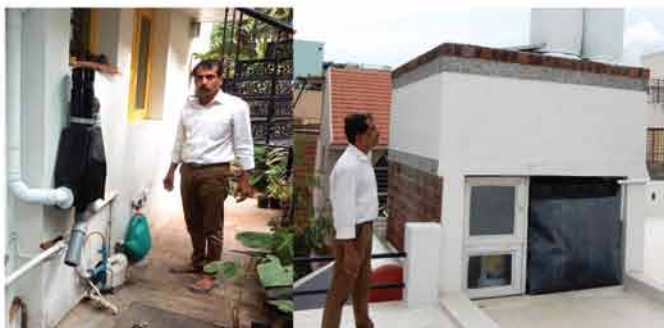
Shivakumar explaining the wastewater usage techniques: (left) water from washing utensils collected in a container to water plants, (right) treatment unit for recycling wastewater from the washing machine
