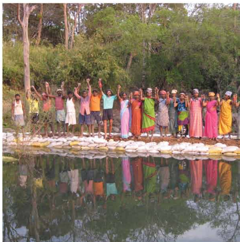
Singh with the residents of Taipadar, after building the makeshift dam
