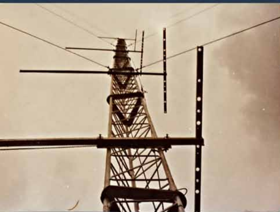
One of the towers used for MONTBLEX, showing its triangular lattice structure
