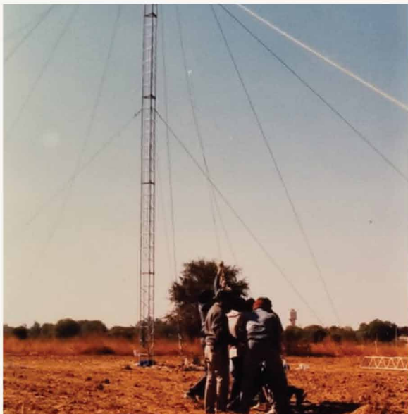
The tower at Jodhpur being erected
