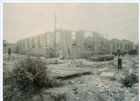
Construction of Electrical lab from northeast corner (1909)
