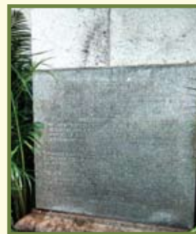
The Corner Stone at the entrance of the Main Building as it exists today
