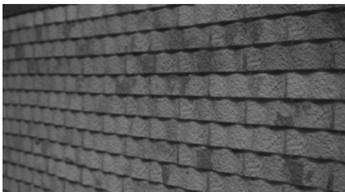
Curved tiles help scatter sound, thus preventing echoes (Photo: Karthik Ramaswamy)
