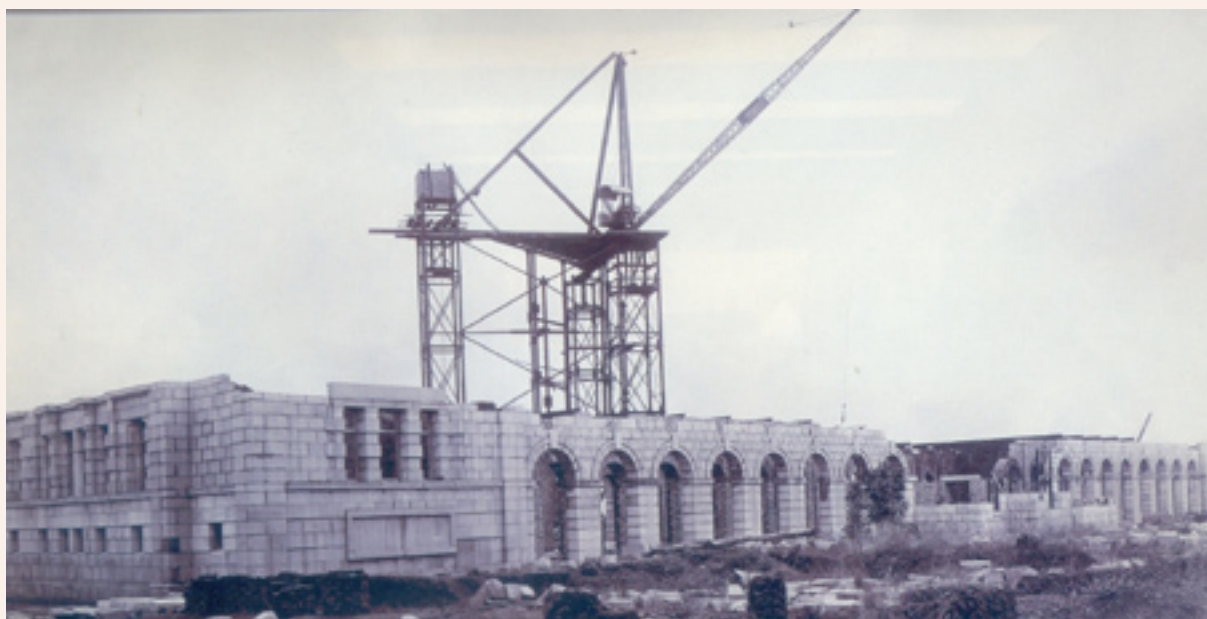
The Main Building under construction
